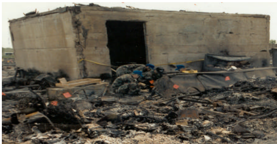
Figure 6.2 FBI photo. Bunker walls were made of plastered cinder blocks.
