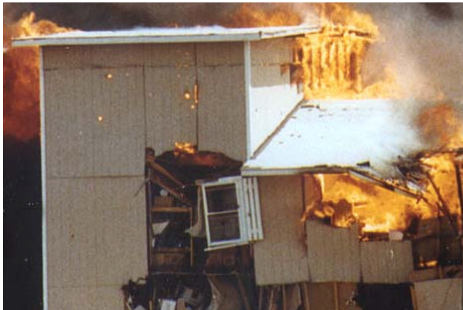
Figure 3.4 FBI ground photo. The Green/White tower on fire. Similar holes as shown here on the third floor allowed flames to emerge out of the cafeteria Black Side wall in the very early stage of the fire, cf. Figure 2.12.
