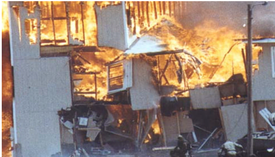
Figure 2.1 FBI ground photo of Green/White tower. The front wall was covered on the external side with wood panels and on the inside of first two floors with drywall (gypsum boards). The tower second and third floor walls had no internal claddings.
