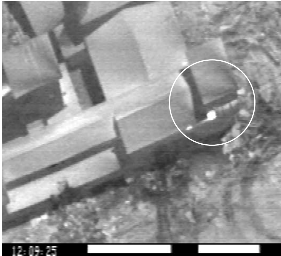
Figure 2.18 FLIR image 12:09:25. A bright heat image in the second floor window immediately to the left of the tower. Heat images also due to heat conducted through second floor tower wall. The wood studs appear as cooler (darker) than the fields between.
